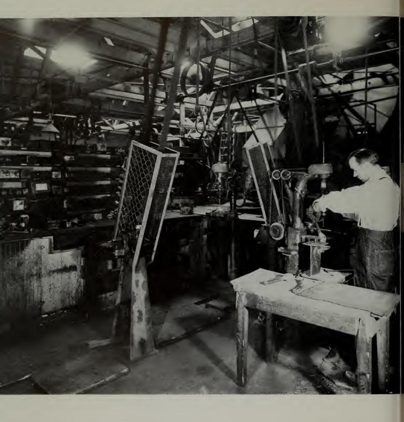
The oil holes are not always the same size. Accordingly, the operator uses a second drill press with a larger drill to perform the same operation shown in Picture 18. This removes the necessity for frequently changing drills.
